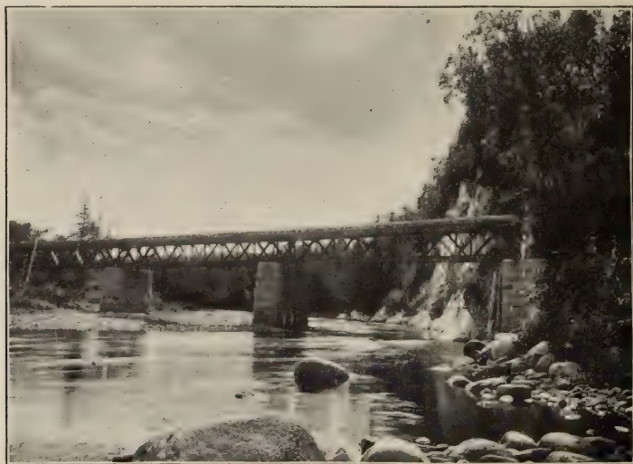
Newfoundland Railway Bridge.
